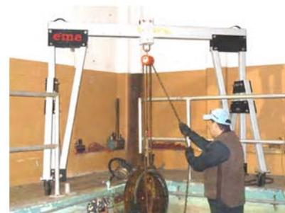
Operator shown lifting defective valve cover
